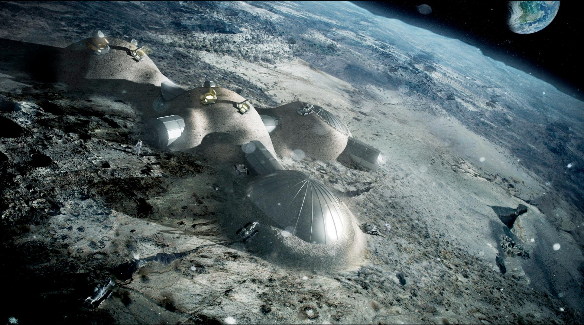
*Setting up a lunar base could be made much simpler by using a 3D printer to build it from local materials. Industrial partners including renowned architects Foster + Partners have joined with ESA to test the feasibility of 3D printing using lunar soil*
