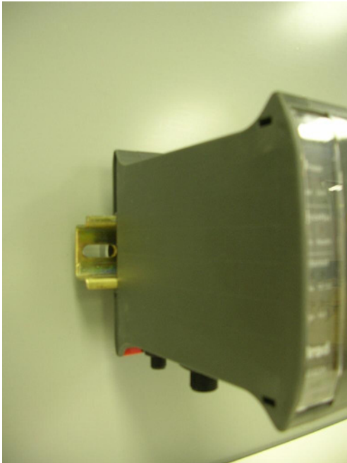
Figure 4: Remote Scanner Installed
